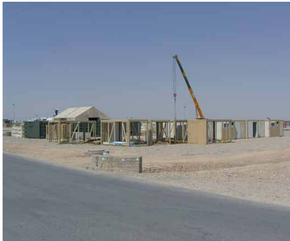
Setup of Z-Containers.
